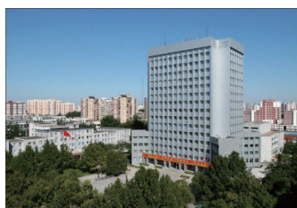
Fig. 1 Main Building in BUPT campus, Beijing
